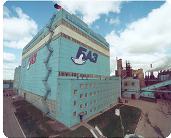
Figure 1: Thus, Bogoslovsky Aluminum Plant made its first and, perhaps, the most complex steps on the way of ASU-GLINOZEM MES system implementation.
